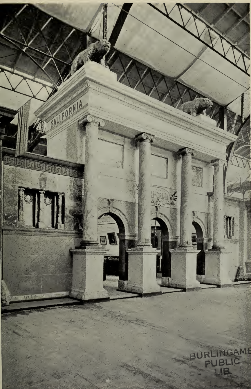
Front of State Mining Exhibit. Facade constructed of marble, granite, onyx, sandstone, and other building stones from California—MINES AND MINING BUILDING. (Page 78.)
